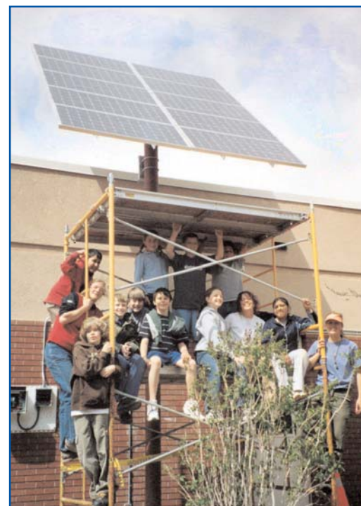
The solar photovoltaic system installed on the Basalt, CO Middle School
