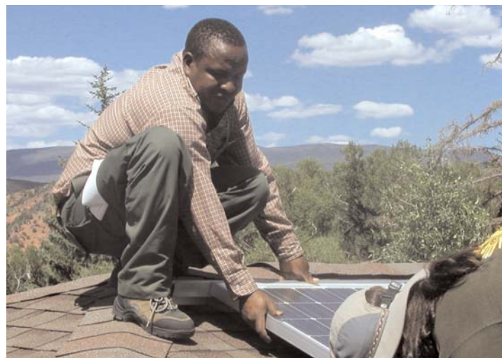
Maina Stanley Gathai installs a solar PV system in an SEI workshop.
