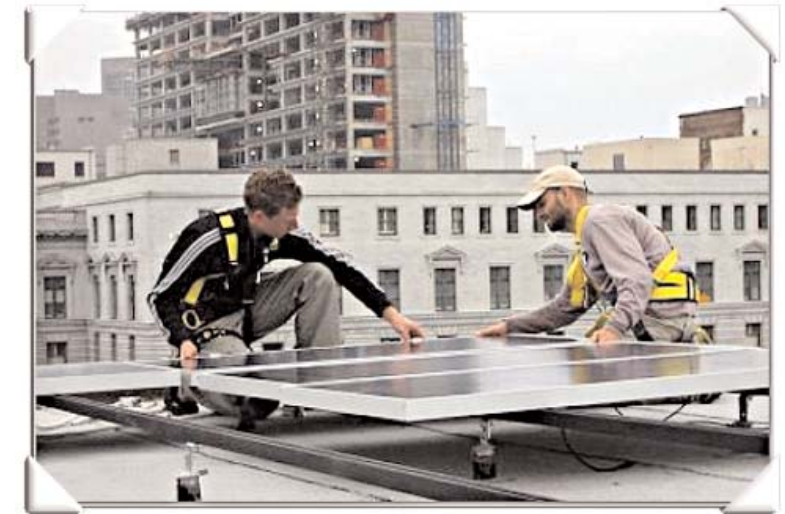
SEI workshop participants install a PV system in San Francisco.
