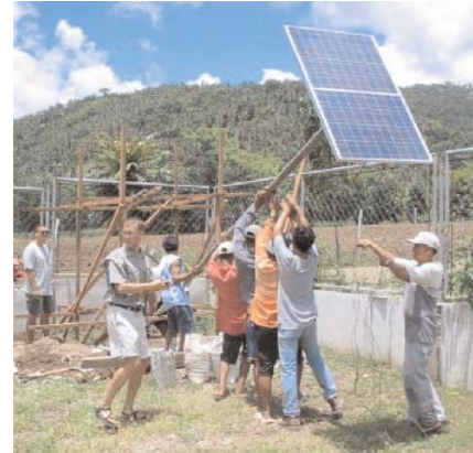
A PV system is installed in the Philippines.
