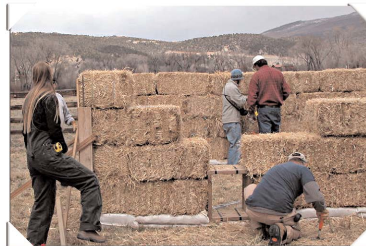
Building a straw bale shed in the Intro to Straw Bale workshop
