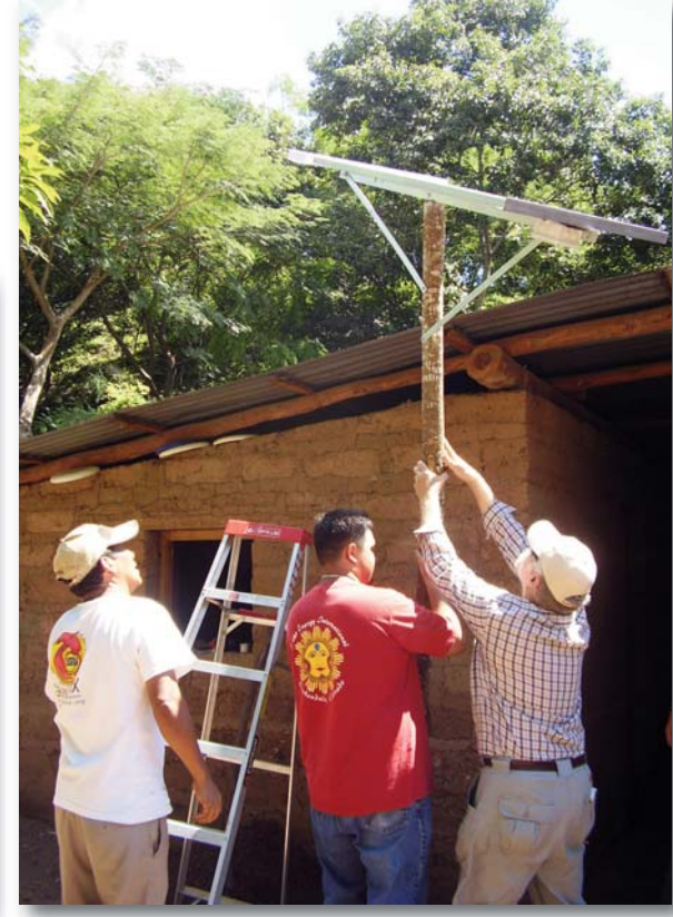
Installing a PV system in the Renewable Energy for the Developing World workshop in Nicaragua ◀
