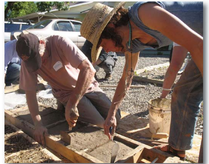
Making adobe blocks in the Designing & Building Natural Homes workshop ▶
