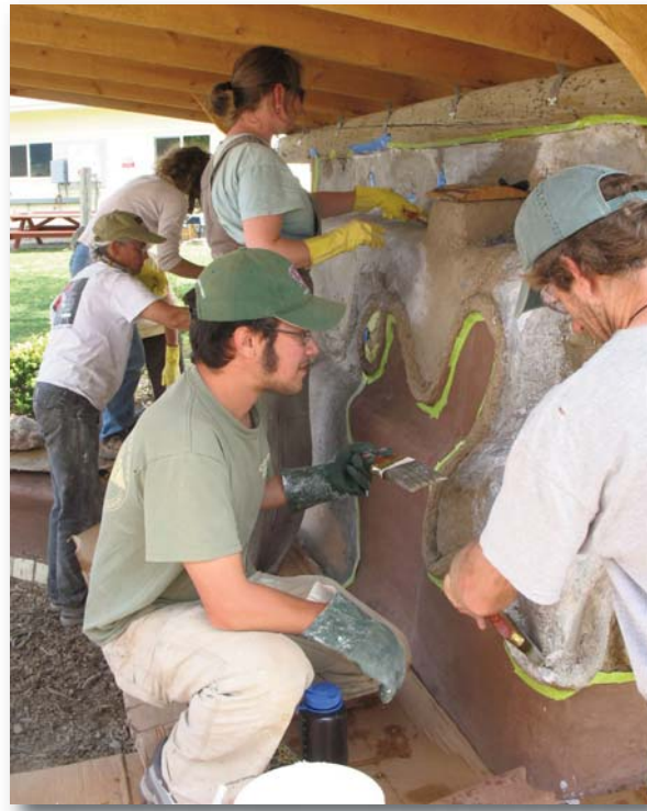
Plastering a wall in the Strawbale Construction and Natural Plaster workshop ◀
