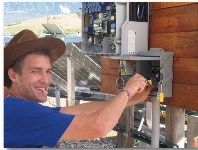
Wiring the power center in the PV Lab Week workshop ◀
