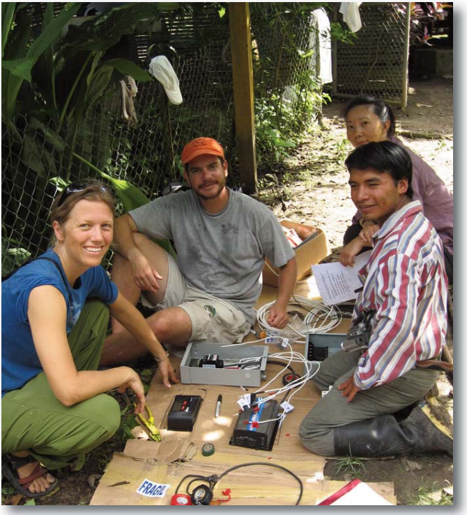
Wiring up the control center for the PV system in Ecuador in the Ecology, Permaculture and RE Workshop ▶
