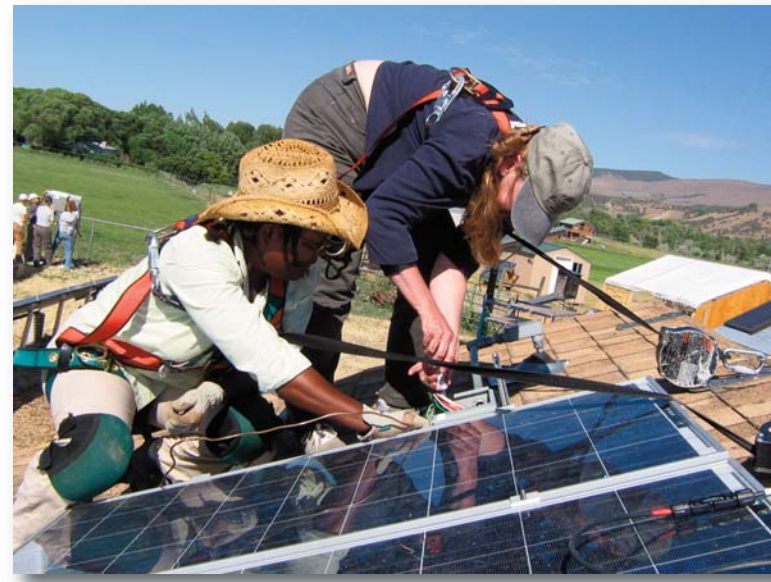
Installing PV modules in the Women's PV Design & Installation workshop ▼
