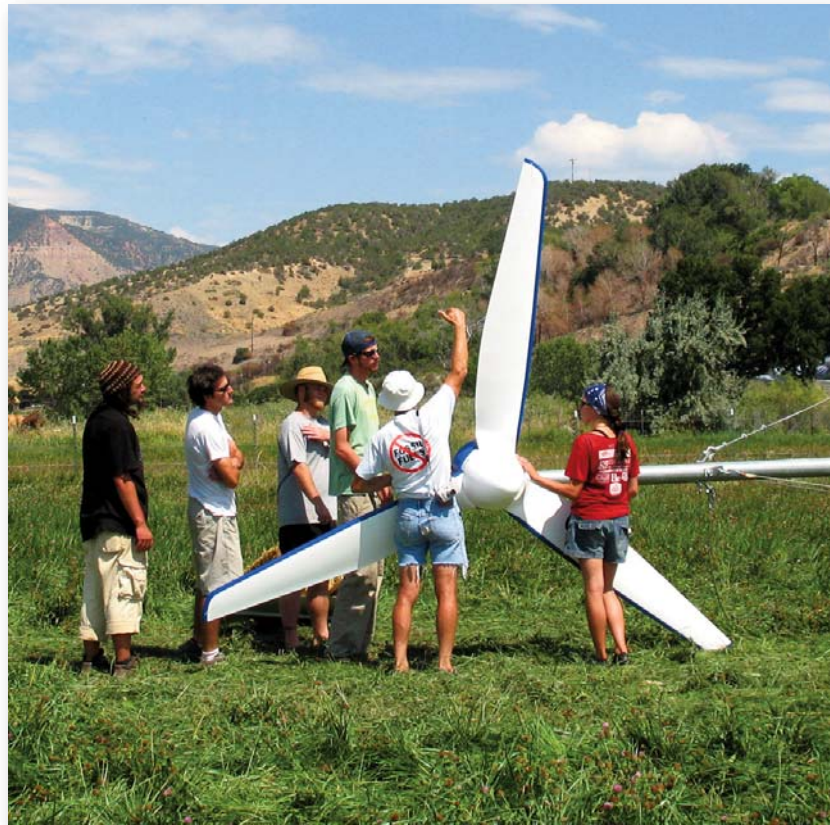
Installing a wind turbine on the Paonia ecocampus
