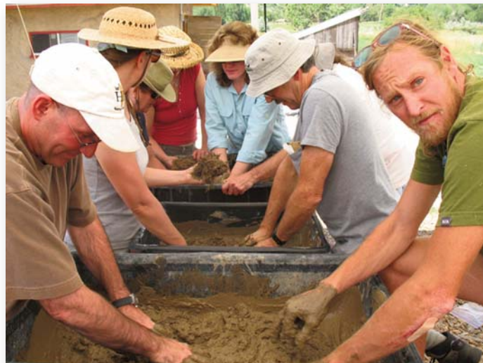
Getting hands dirty with natural plaster
