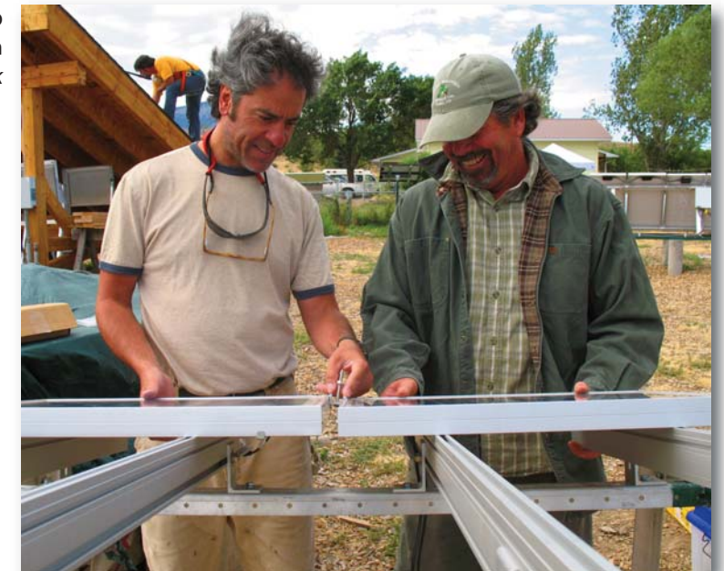
Wiring up modules in PV Lab Week
