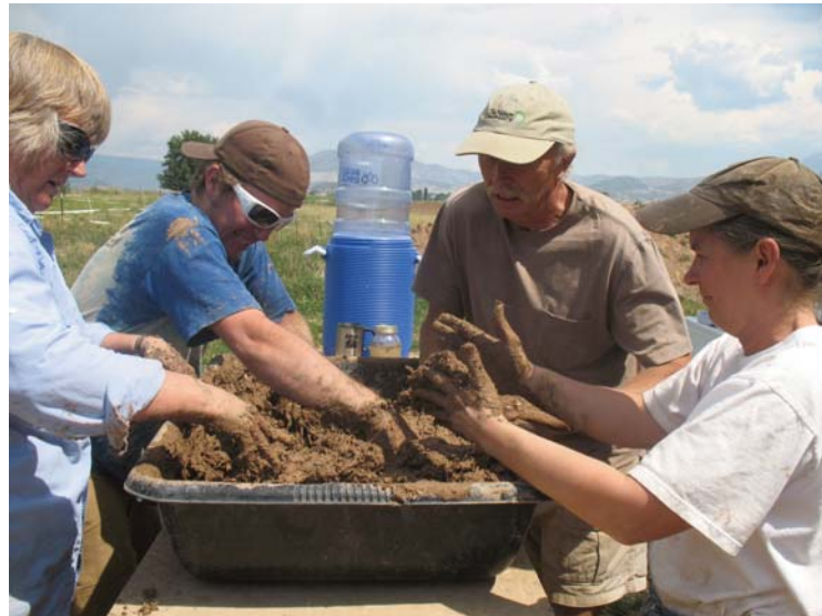
▲ Making natural plaster in the Strawbale Construction and Natural Plaster workshop.
