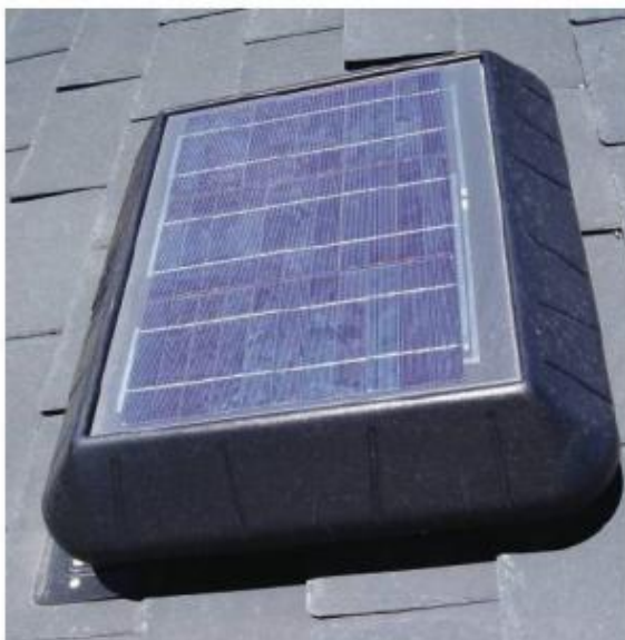
Figure 4.3: The PV module provides power for the attic fan; when there is lots of sun—and presumably lots of heat in the attic—the PV module directly runs the fan.
