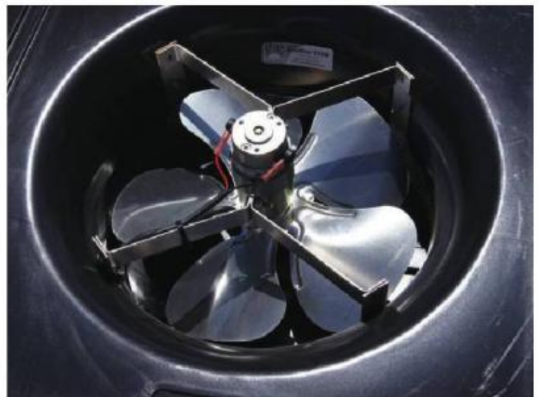
Figure 4.3: The PV module provides power for the attic fan; when there is lots of sun—and presumably lots of heat in the attic—the PV module directly runs the fan.
