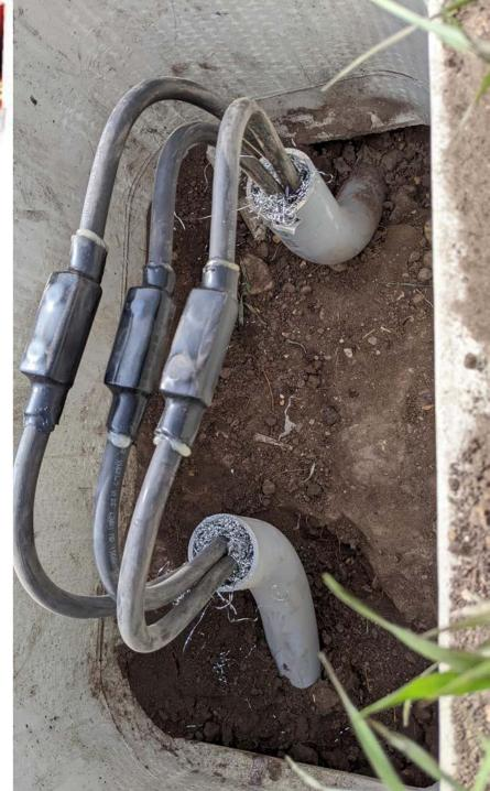
Plugging unused holes in electrical boxes is a **NEC** code requirement NEC 110.12(A)
