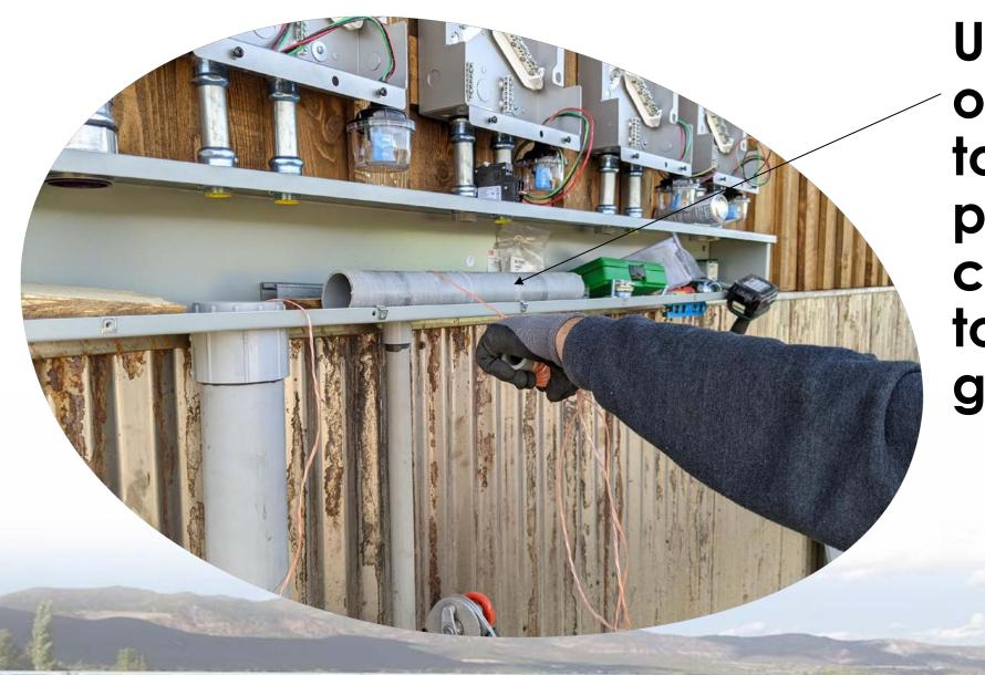
Use a piece of conduit to assist pulling wire connected to wire gutter
